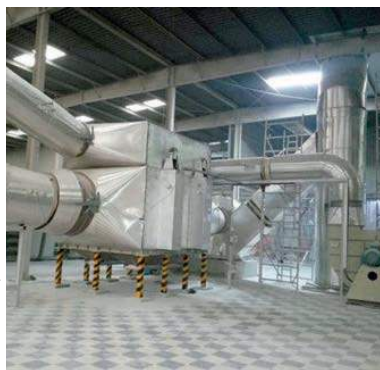
Econotherm's heat pipe heat exchangers can supply combustion air pre-heaters with recovered heat that is otherwise lost.
