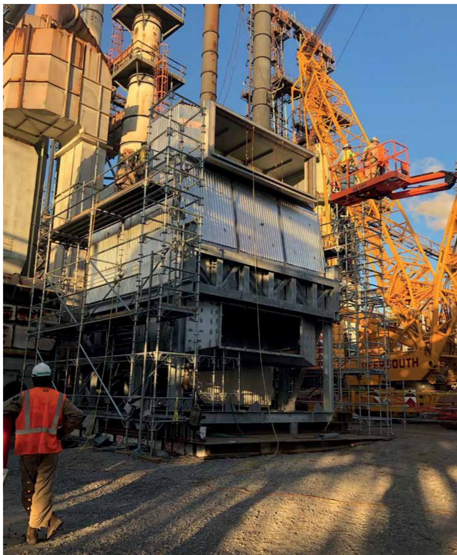
The pipes in heat pipe heat exchangers provide operators with greater reliability in that they can expand and contract without applying stress to casing. This, in combination with thicker walls, reduce erosion and can handle hot and highly acidic gases that are typical in fertilizer production plants. Photo credit - Econotherm
