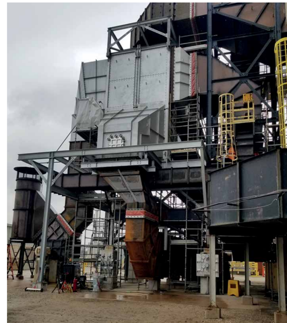
Fertilizer operators can recover exhaust gas coming out of gas-fired heaters using a heat pipe heat exchanger and insert it back into the heater to reduce natural gas costs. The process is similar to waste heat recovery methods already being demonstrated via similar fired heaters in oil refineries. Photo credit - Econotherm
